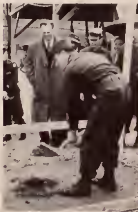
Gen. Lyman L. Lemnitzer, U.S. and U.N. Commander-in-Chief in the Far East, breaks ground on CCU site for Eighth Army Memorial Chest Hospital (Severance), on April 23, 1955.
